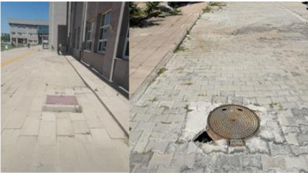
Figure 6. Infrastructure facilities covers
