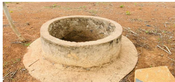
Picture 3. Irrigation wells used in Founia county
