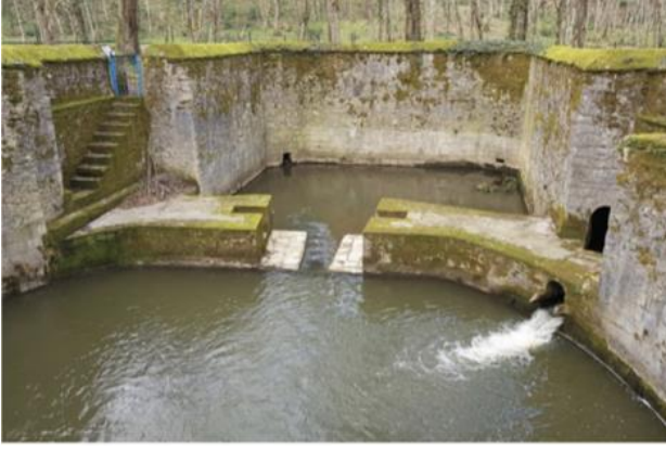
Figure 14. Water Tanks (Dumanoglu, 2020).
