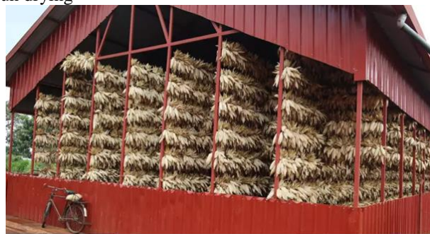
Picture 3: Image of dry shelter
