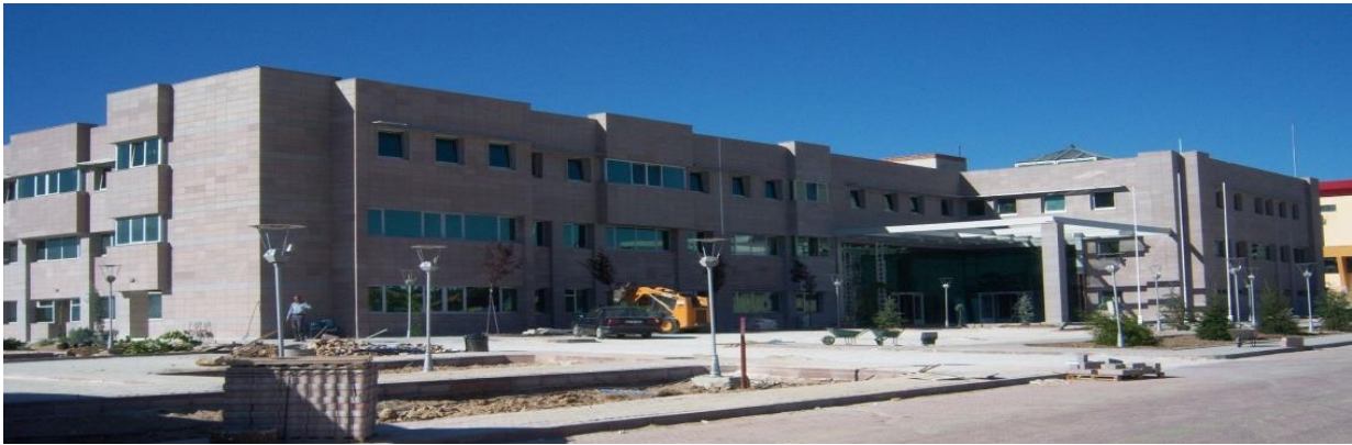
Figure 9. Mechanically assembled andesite cladding exterior facades (Image belongs to the authors)
