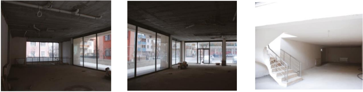
Figure 1-2-3. General Views of Office Floors
